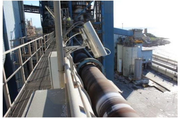
RKS300 system in operation
